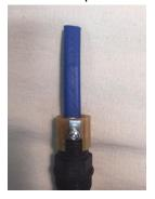
8. Place a layer of  $\frac{1}{2}$  (13mm) glass fiber tape around the cable flush with the top of the Strain Relief. For **PGH** – cut and remove the inner jacket and black fibers down to the top of the tape, exposing the bus wires.
